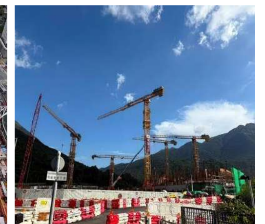
Construction of Public Housing Development at Tung Chung Area 42
